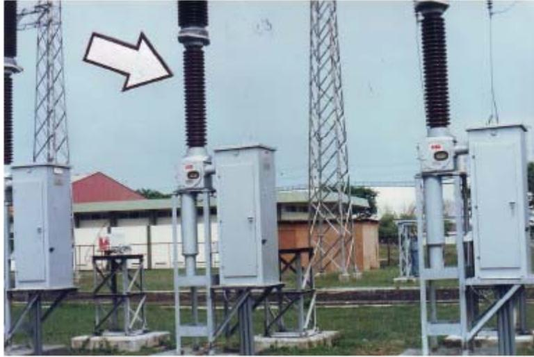
Gambar 3.5 Circuit Breakers
