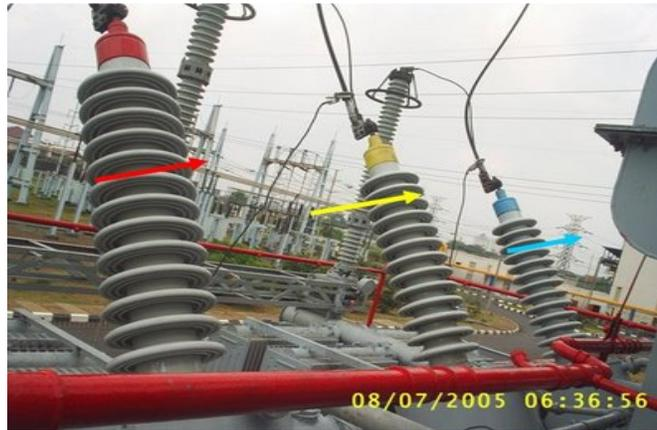
**Gambar 5. 15d. Bushing trafo daya**
