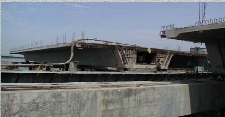
Gambar 2.49 Kerangka acuan (form work) gelagar kotak
